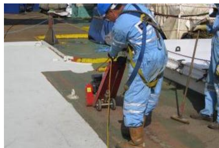
Coating & corrosion removal
